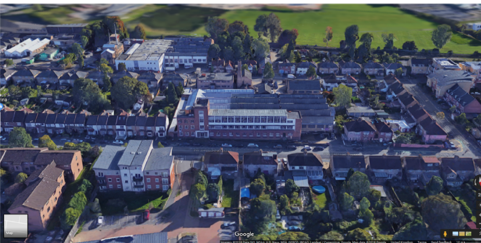
View of site from the north
