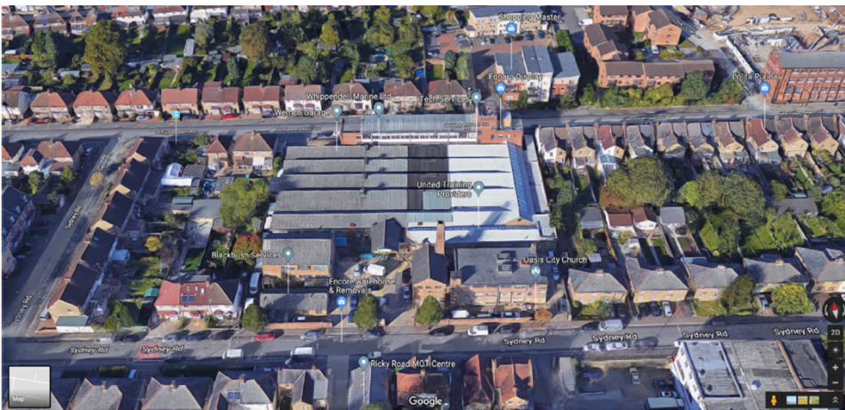
View of site from the south
